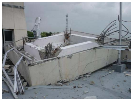
Collapse and falling of a penthouse (塔屋の崩壊・落下)
