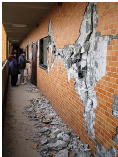
Damage of non-structural wall (非構造壁の損傷)
