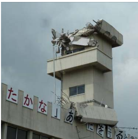
Collapse and falling of a penthouse (塔屋の崩壊・落下)
