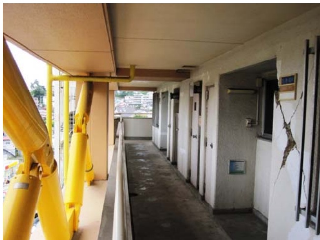
Damage of non-structural walls of a building retrofitted with oil dampers (オイルダンパーで補強された建築物の非構造壁の損傷)
