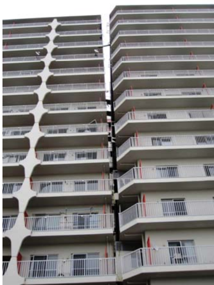
Tilting of a building (建築物の傾斜)
