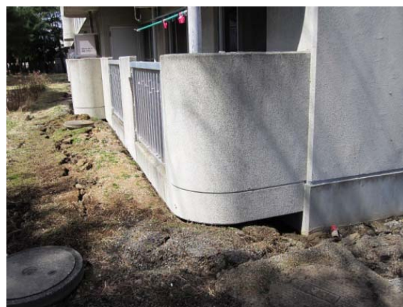
Settlement of a building (建築物の沈下)
