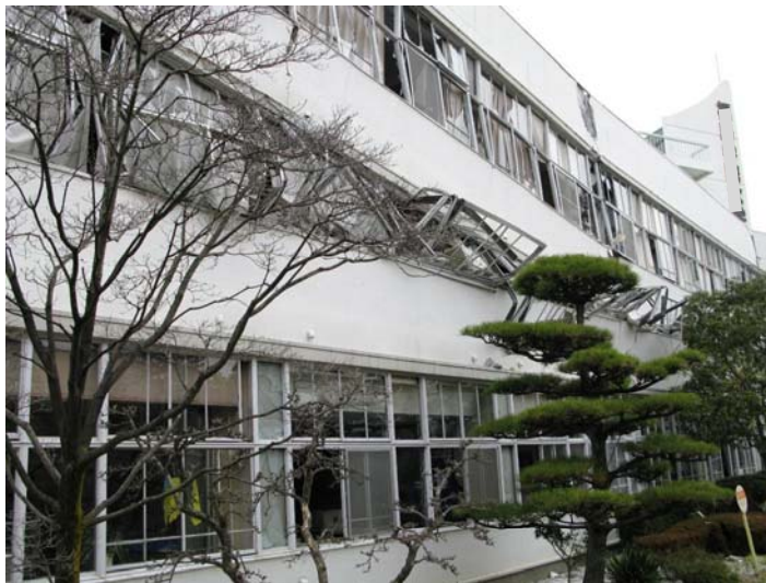
Collapse of middle story (中間階の層崩壊)
